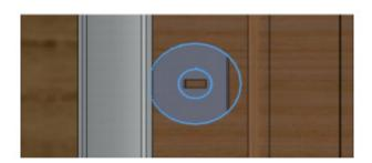
4. Once the lock is placed in the centre of the machined frame, use the 3.5mm drill bit and drill pilot holes in the top, bottom, and centre of the hinge. The stainless-steel tip needs to be within 0.5mm of the top of the frame, if not, adjust the 25mm hole to suit.
